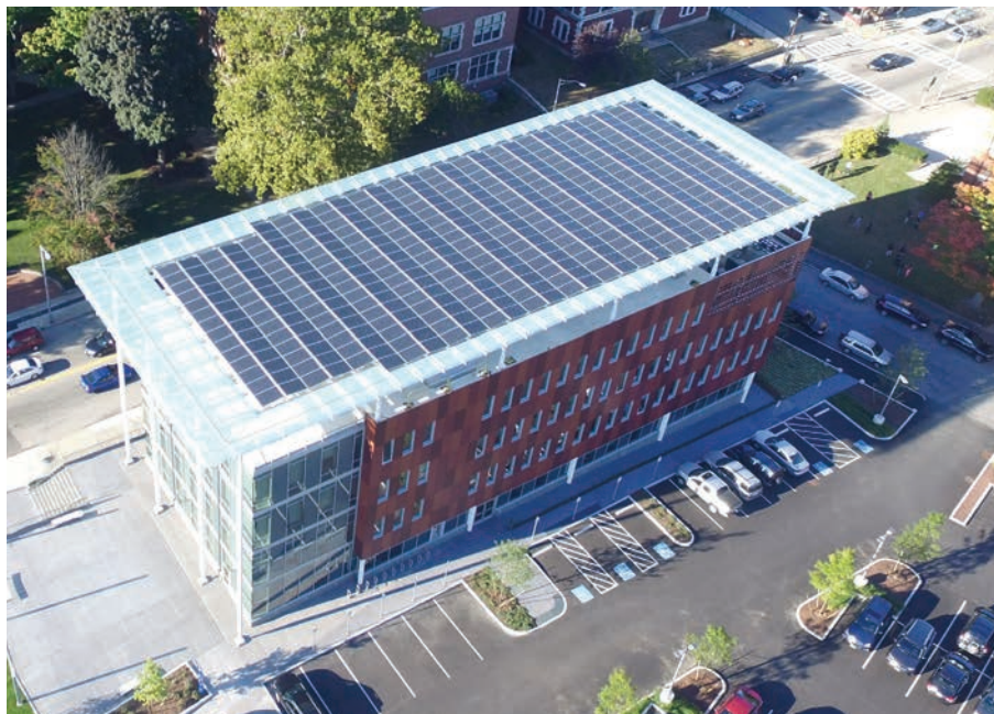
Area constrained Solar Design Associates used a dual-tilt mounting system at Clark University's Alumni and Student Engagement Center to maximize ground-cover ratio, total system capacity and energy yield per unit of area.
